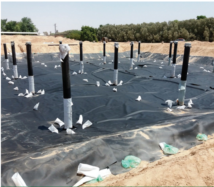
Figure 1: Sealed bottom surface of the lysimeter with the right slopes for each tree basin before filling with soil
